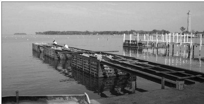
The old L-shaped dock has been removed, the area was dredged to provide proper depth, three steel cribs have been set, and connecting I-beams are in place. Welding work will continue, and the concrete in front of the pavilion will be raised 4 inches. Concrete will be poured on top of the cribs in the spring, followed by all of the finishing touches to be completed in time for the 2005 boating season. You can view the construction progress at [www.pibyc.org](http://www.pibyc.org).
